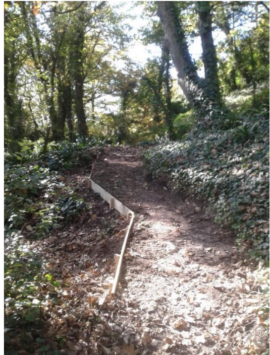
Retaining boards to enable levelling/widening of path and reduce erosion
